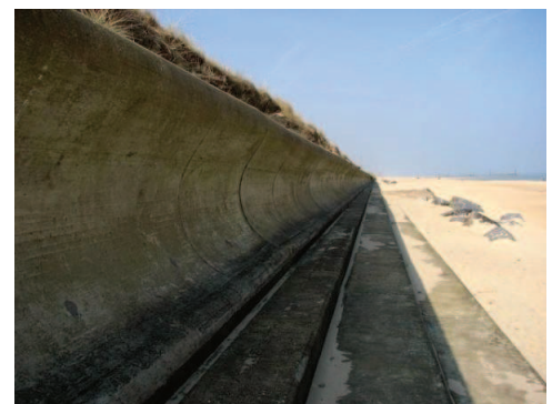
A concrete seawall along the beach.
