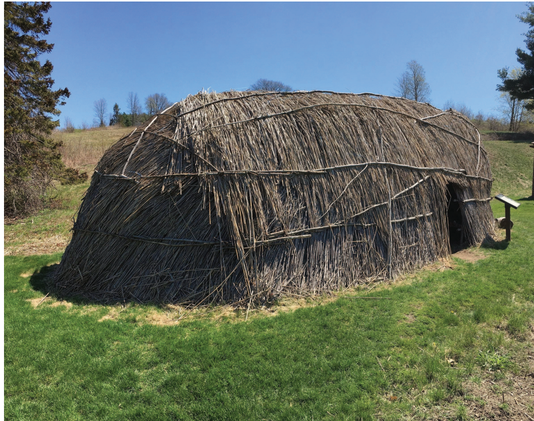
Wetu are built from natural materials found in the Northeast region of the United States, such as elm trees and cattails.
