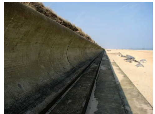
A concrete seawall along the beach.
