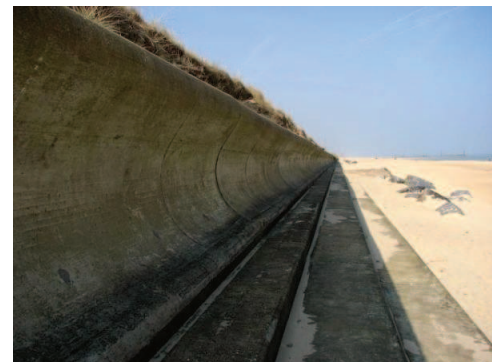
A concrete seawall along the beach.
