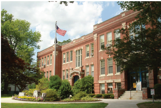
Town Hall in South Hadley, Massachusetts
